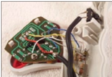
Photo 8: Final controller connections.
